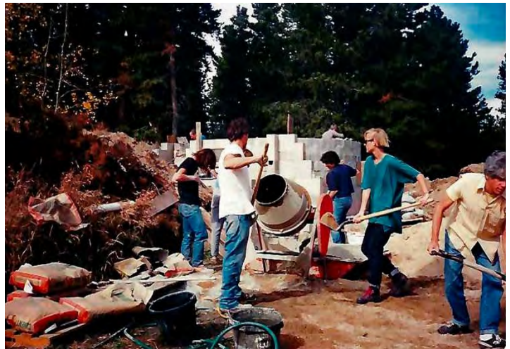
photo: volunteers mixing and pouring the walls, from Jeff Combelic
